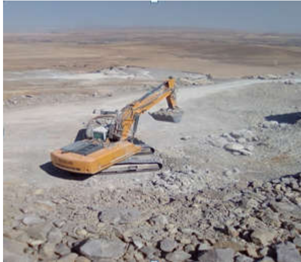
Pelle excavatrice LIEBHERR R54C
