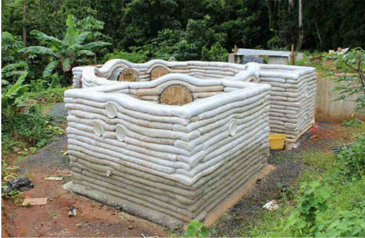
This is one of several eco-houses under construction at Plenitud Eco-Iniciativas in Puerto Rico.
