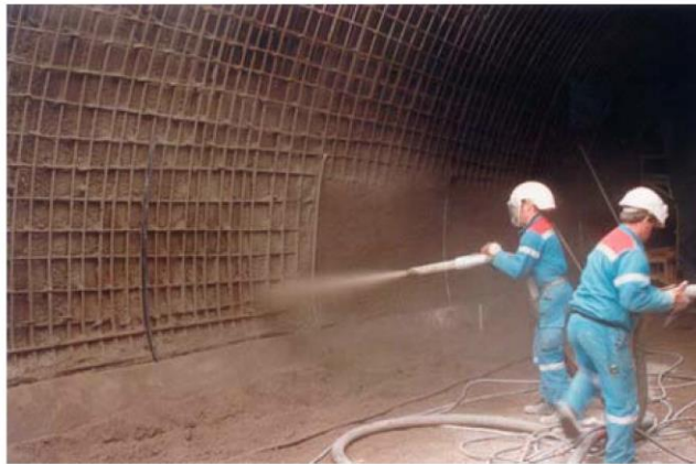
Figure 1: Projection de béton
